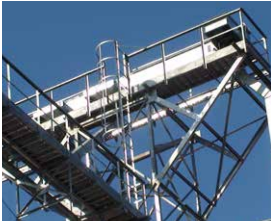
— Photo of ladder from eave platform to catwalk
