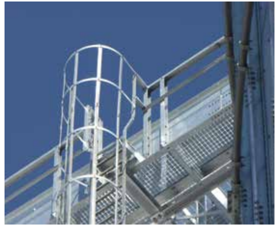
— Photo of front landing to access catwalk
