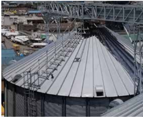
— Photo of roof ladder
