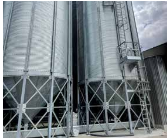
— Photo of ladder from ground to eave platform of FC silos
