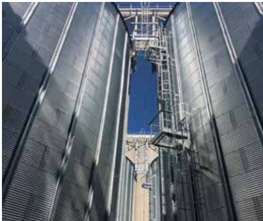
— Photo of ladder from ground to eave platform of FP silos
