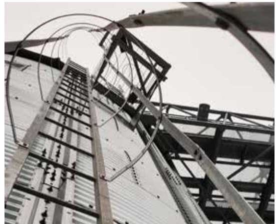
— Photo of ladder safety cage
