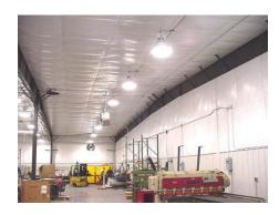
Sentinel's Thermal Efficiency System consists of a network of fastened steel straps supporting large sections of high-strength vapor barrier fabric, each designed to fit a specific ceiling or wall section. Various insulation types can then be installed on the ceiling system from either the top or underside to obtain virtually any desired insulation R-Value.
