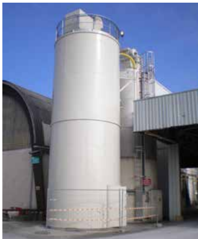
Single block round silo with skirting
